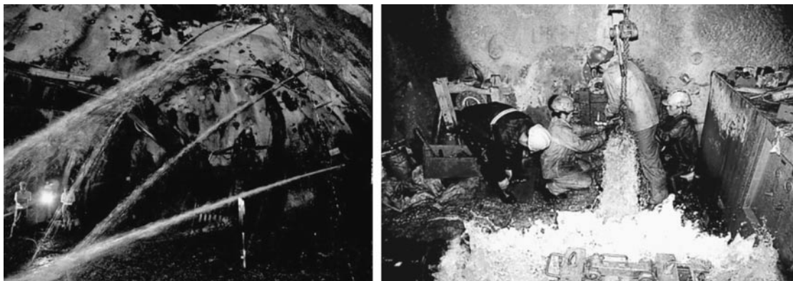
Photo. 1 Groundwater Condition in the Hsueshan Tunnel
